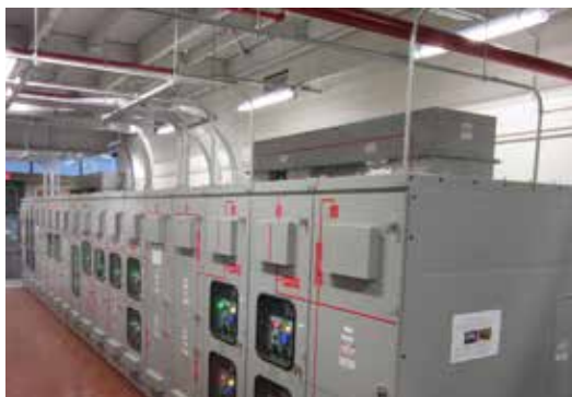
▲ LEFT TO RIGHT: New 4,160 V distribution switchgear for the emergency power distribution system was installed. Exterior of new generating plant near completion.
