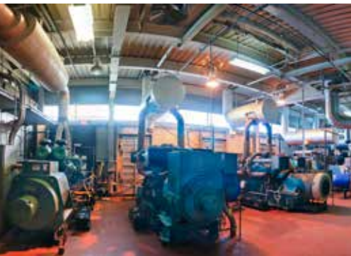
▲ LEFT TO RIGHT: Interior view of Sunnybrook's existing generator plant. Four new 2 MW - 4,160 V and one new 750 kW - 600 V diesel generators were installed. The existing generator plant was dismantled in two phases and the new plant constructed in two phases.
