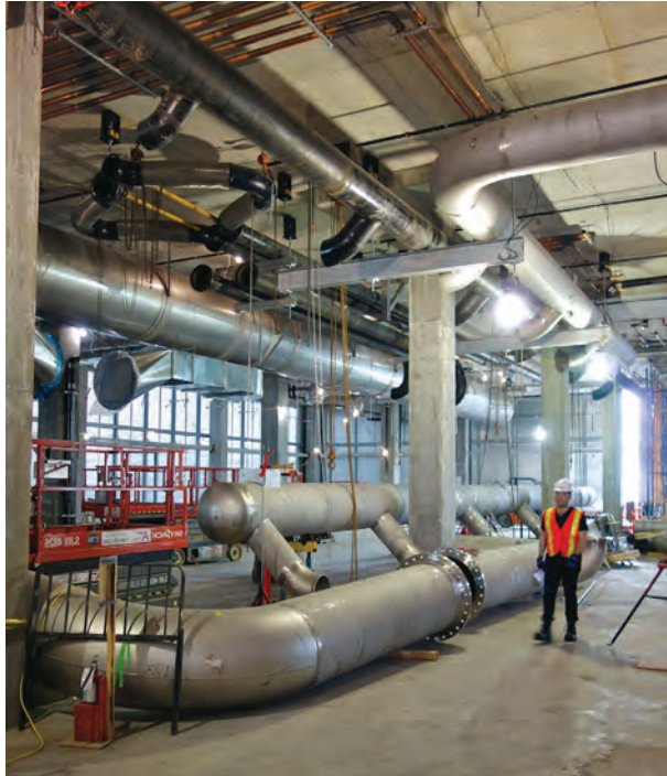
Stainless steel condenser water header located in the plant room on the 17 th floor of the outpatient block.
